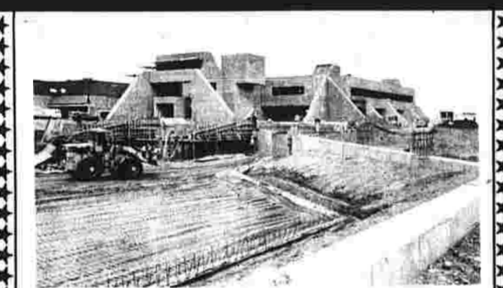
The J.C. Penney Distribution Center.
